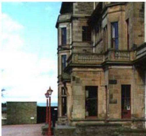
Craiglockhart facility in Edinburgh, the psychiatric hospital where Wilfred Owen met Siegfried Sassoon
