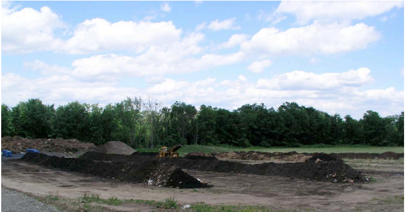
Figure 1.1 The Cayuga Compost facility that serves the greater Ithaca area. Started in early 2006, the facility now has several windrows that can attain temperatures as high as 70C (160F).
