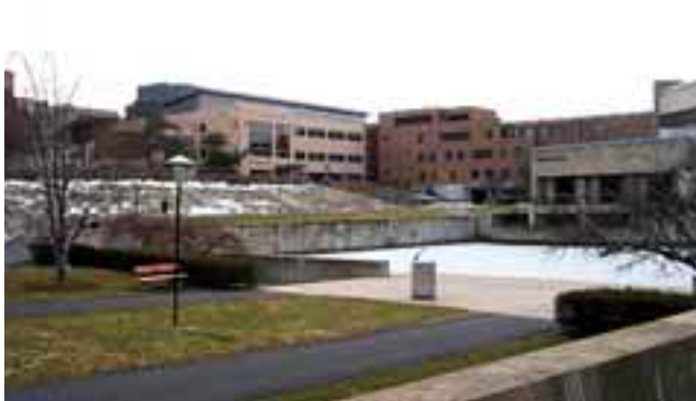
Before: Existing Rip-Rap Wall at Hill Center
