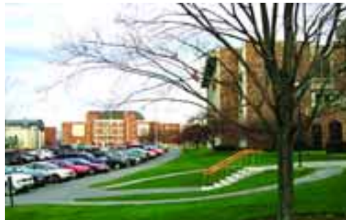
Before: Existing parking north of Job, site of future Main Street
