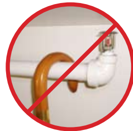
Items hung from Ceilings or Pipes
