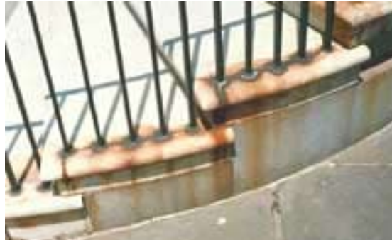
e. Care must be taken to ensure that replacement and historic materials are chemically compatible.
