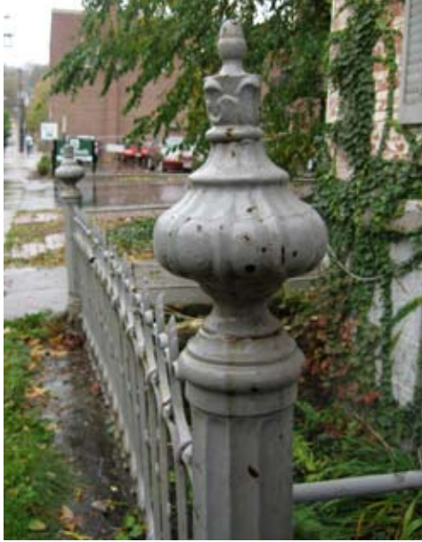
Cast iron fence post on Seneca Street.
