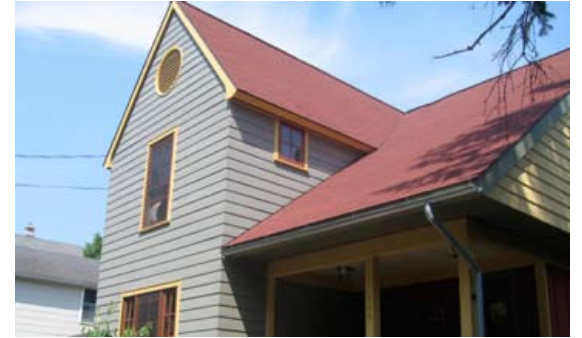
g. New construction should compliment but not replicate its historic surroundings.
