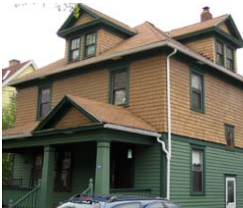
Painting new gutters and downspouts to match the paint scheme would help make them less obtrusive.
