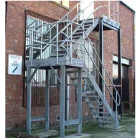
Fire escapes should be located at the side or reare of the building, due to thier visual impact on the building.
