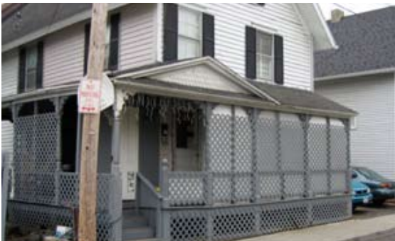
c. Don not use replacement materials that are not sympathetic to the rest of the building.
