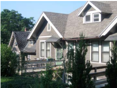
Carriage houses converted to apartments on University Avenue.
