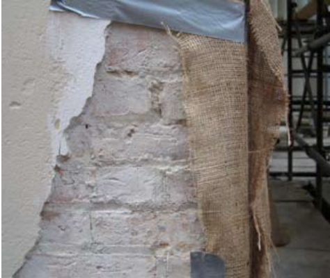
Careful restoration work at the Clinton House, repairing the stucco.
