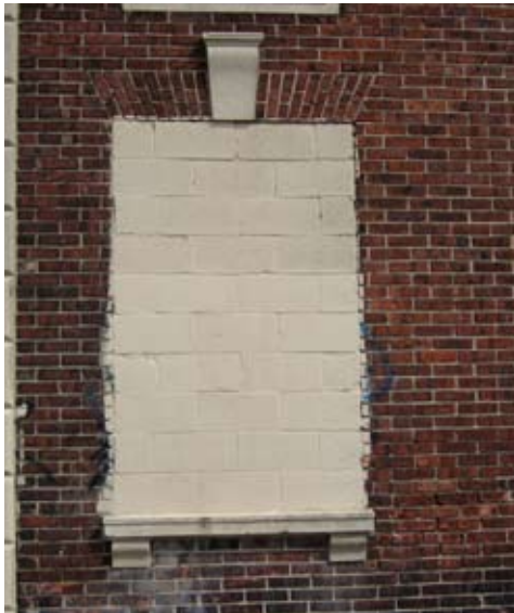
Historic windows should not be blocked up
