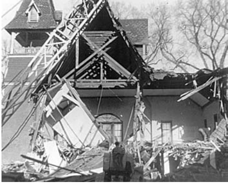
Demolition of the Tabernacle Baptist Church, Utica Street, circa 1964.
